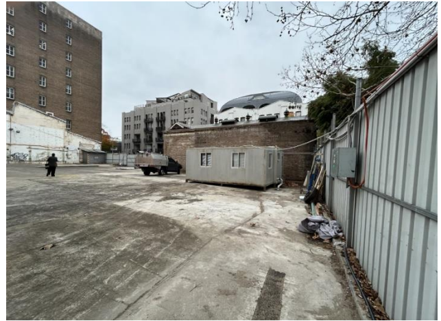
Figure 29 View northwest detailing in ground drainage connections and hardstand concrete,
