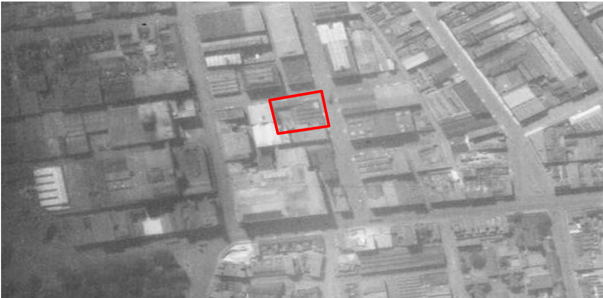
Figure 17 – Aerial photograph dated to c.1928. Approximate location of the subject area as indicated in red.
