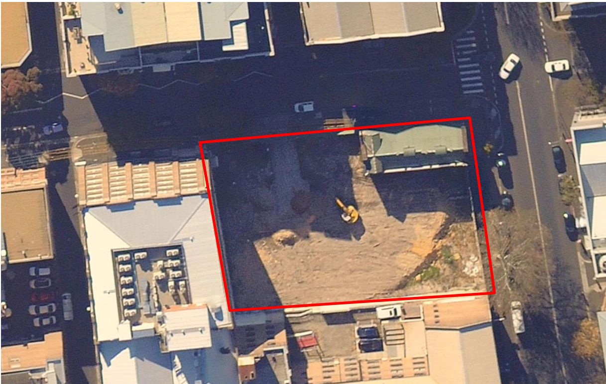
Figure 21 Aerial photograph 2010 detailing the preparation works for the extant structures within the subject area and addition of fill layer.
